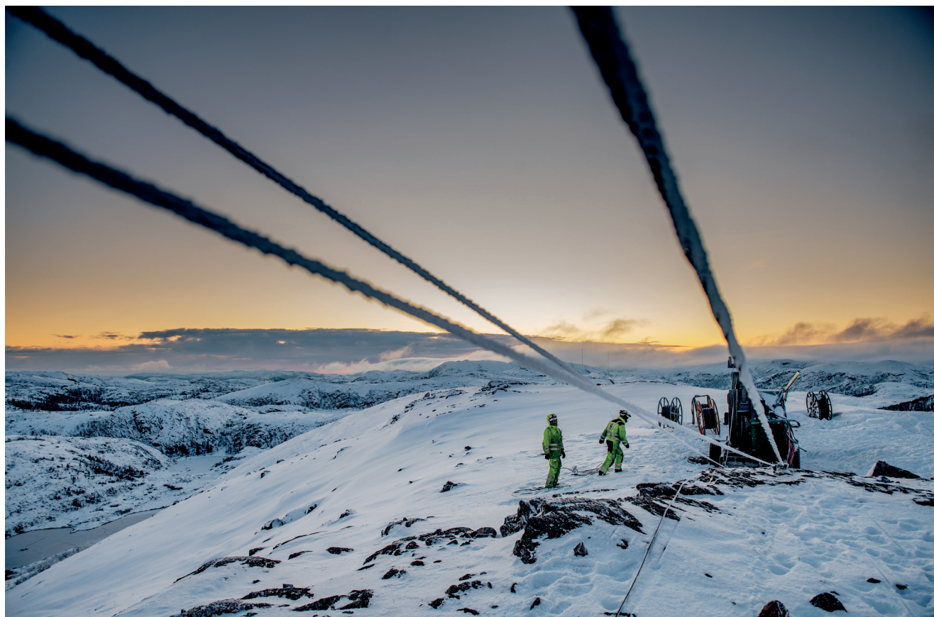
Grid installation at Haraheia. Photo: Ole Martin Wald
