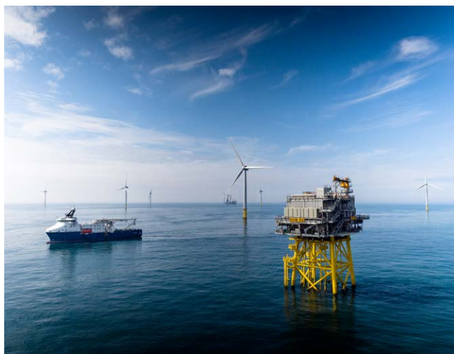
Dudgeon Offshore Wind Farm
